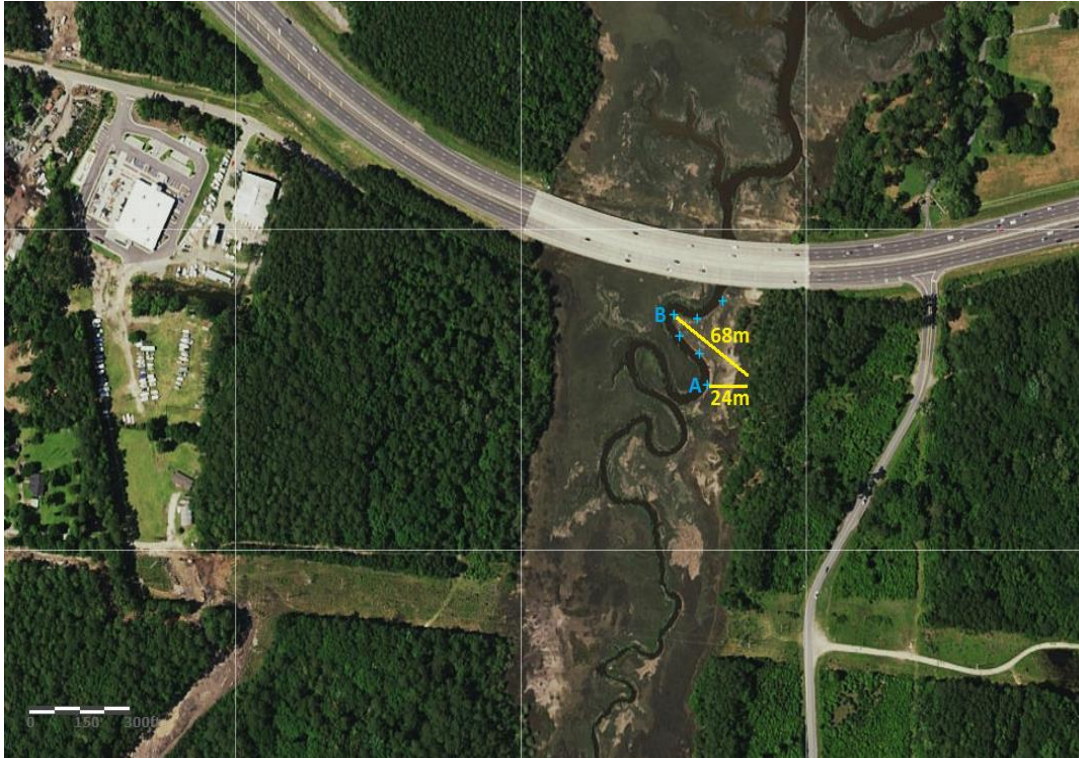
Figure 2.1. A salt marsh/tidal creek system surrounded by suburban development in Okatie Creek, SC, where the width of the marsh (between the forest-marsh boundary and the creek bank) varies along a single marsh section. Point A shows a marsh width of 24 m and an upland of 5600 m; Point B shows a marsh width of 68 m and an upland width of 5600 m.
